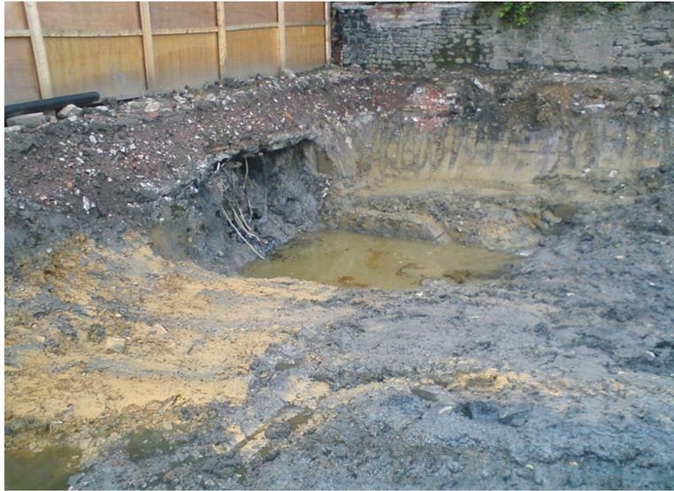
Figure 25.32: Soil contamination caused by underground storage tanks containing tar. (8)
