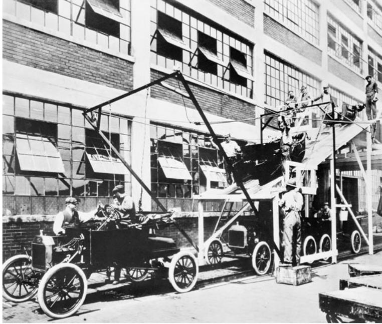
Figure 6.24: Part of a Ford assembly line.
