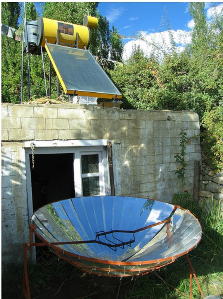
Figure 4.12: A solar cooker and a solar water heater in India. The solar water heater is on the roof of the building. The solar cooker is the silver dish in front of the building.
