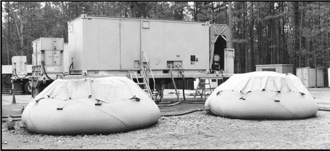
Figure A-3. Reverse osmosis water purification unit
