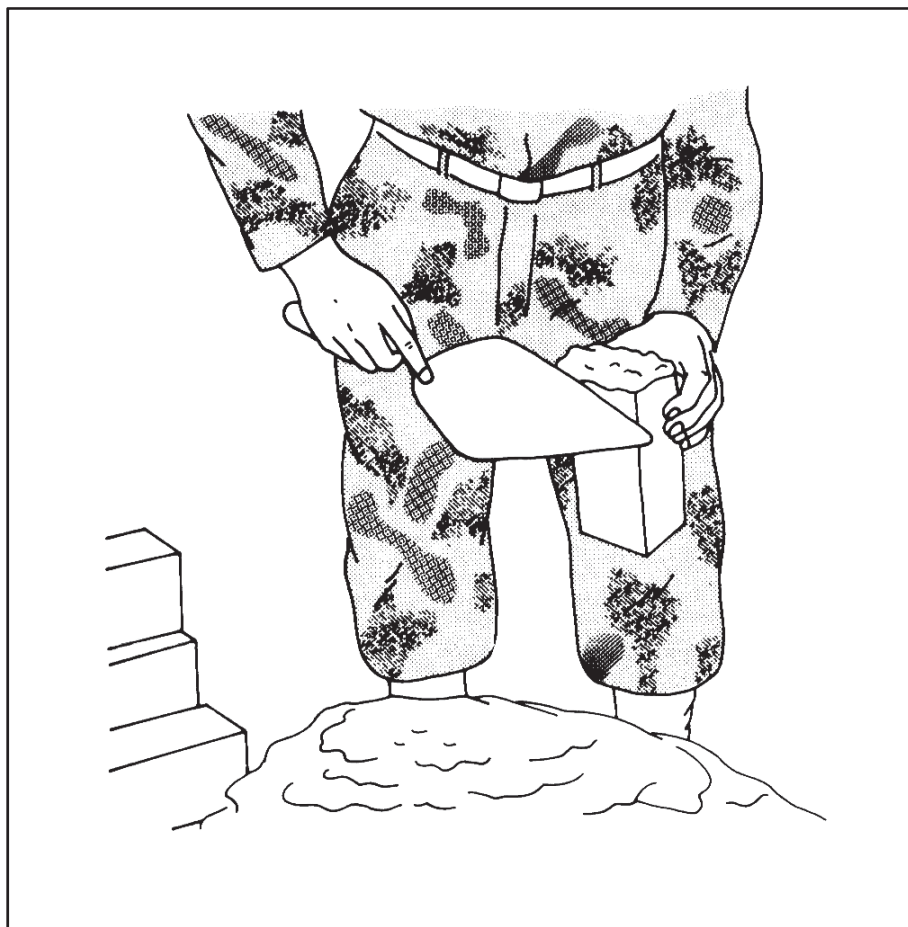
Figure 9-10. Proper way to hold a brick when buttering the end
