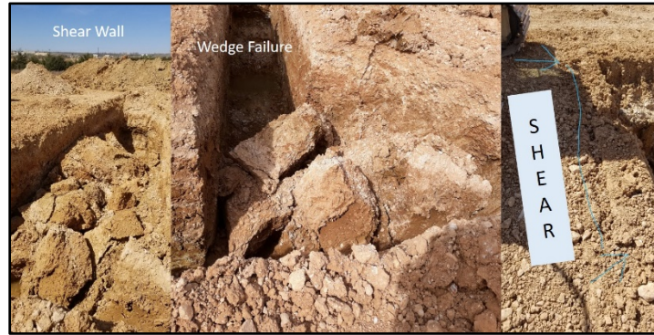
Figure 4-3. Trench failures
