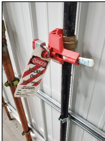
Figure 3-4. Gate valve
