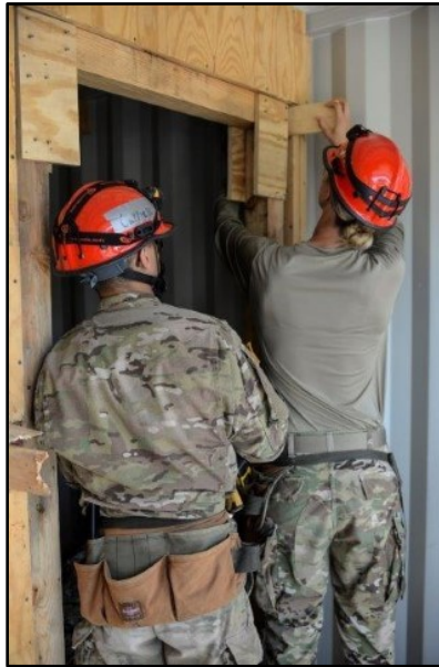
Figure 5-6. Door and window shore
