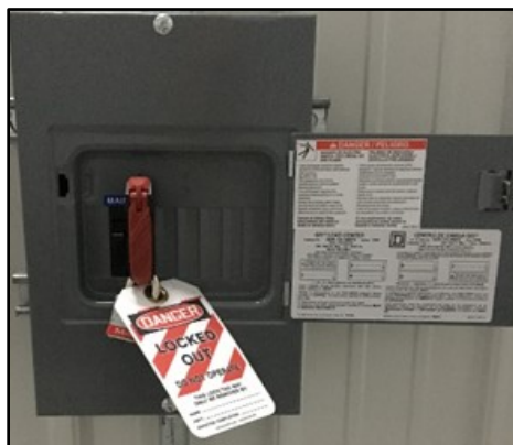
Figure 3-3. Circuit breaker
